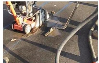
Wet-vac used to collect saw-cutting slurry
