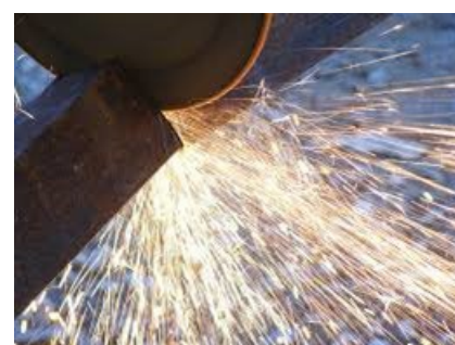
Hot works during a TOBAN need to comply with an exemption
