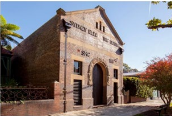
Ausgrid S170 heritage substation. Also, State heritage listed
