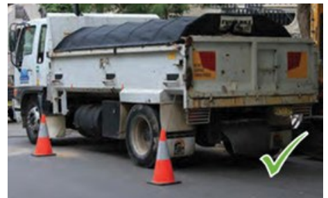
Cover loads to prevent pollution
