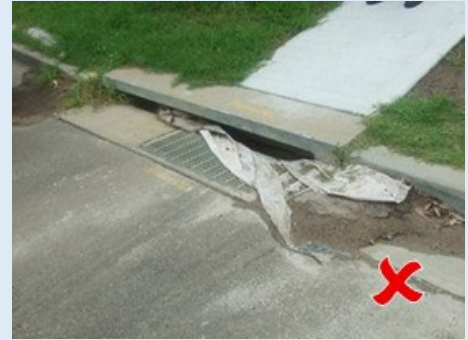
Regularly inspect and maintain erosion and sediment controls
