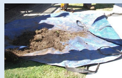
Spoil temporarily placed on tarp to contain spoil and assist clean
