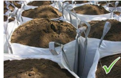
Bulk storage bags help contain materials
