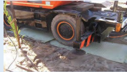
Temporary construction mats help minimise ground disturbance
