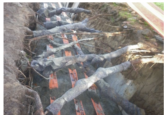
Where roots are exposed for extended periods of time (>24 hours), wrap larger roots (> 50mm diameter) in jute mesh or hessian and keep moist
