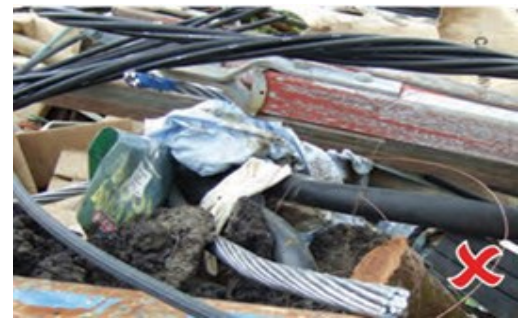
Segregate waste to avoid cross contamination Example of poor waste segregation
