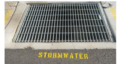
Check whether nearby drains go to stormwater, sewer or an oil containment tank
