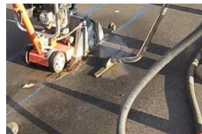
Wet-vac used to collect saw-cutting slurry
