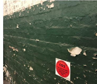
Lead paint on substation wall
