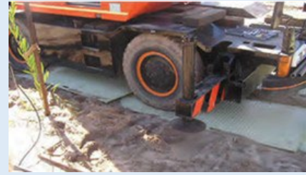
Temporary construction mats help minimise ground disturbance
