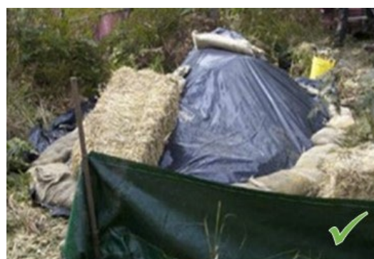
Correctly store ASS to minimise exposure to the air
