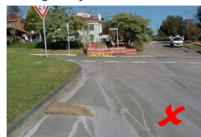
Saw-cutting slurry has not been contained effectively
